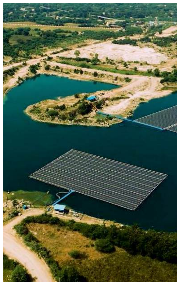
Site - Floating Solar Plant - Udaipur
