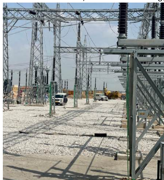
Under Construction Pooling Sub Station, Nokh Jaisalmer
